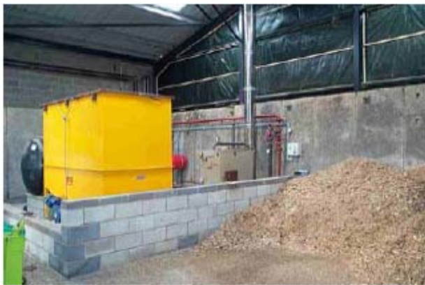
Figure 2. A Veto (80kW) wood chip boiler heating a farmhouse, two cottages, a café and business units
