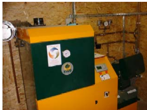
Figure 3. A Vigas (25kW) log boiler, suitable for a 4 bed property (size of medium sized fridge)
