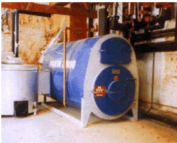
Figure 2. A Veto (80kW) wood chip boiler heating a farmhouse, two cottages, a café and business units
