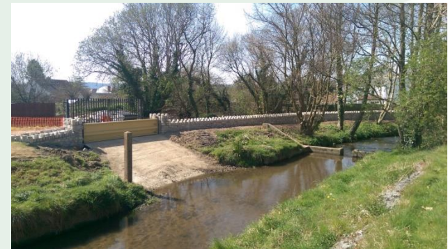
Flood Defence Wall – Phase 1 of Axminster Flood Defence Scheme
